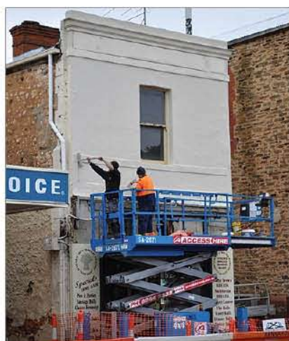
A. Painting of the facade after demolition of the awning and surface preparation.
