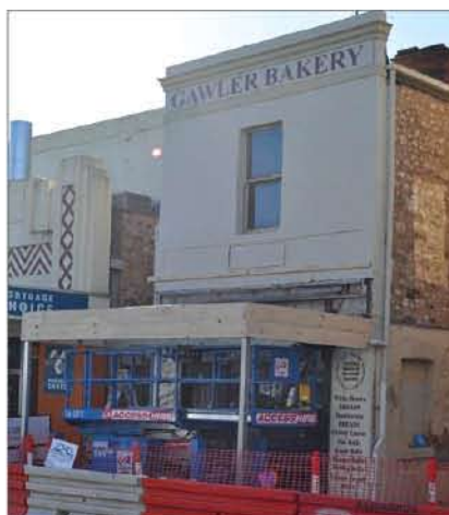
B. Signage (top) and Awning Framework Installed
