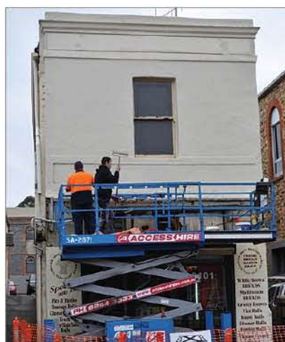
A. Painting of the facade after demolition of the awning and surface preparation.
