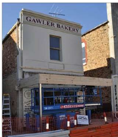
B. Signage (top) and Awning Framework Installed
